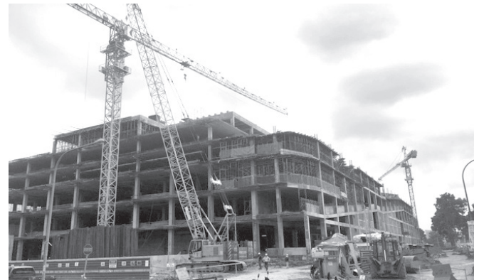
AEON shopping complex @ Jln TAZA under construction
