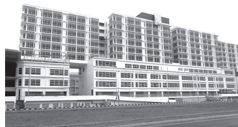
Newly completed SOVO at Bintulu Paragon
