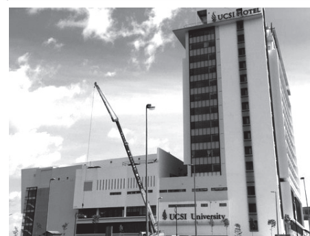
UCSI Hotel at Kuching Isthmus, nearing completion
